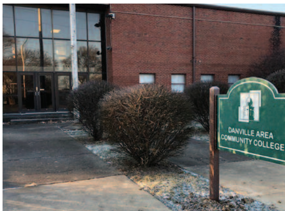
Entrance to the U.S. Army Reserve, DACC's future home for expanded healthcare-education programs.
